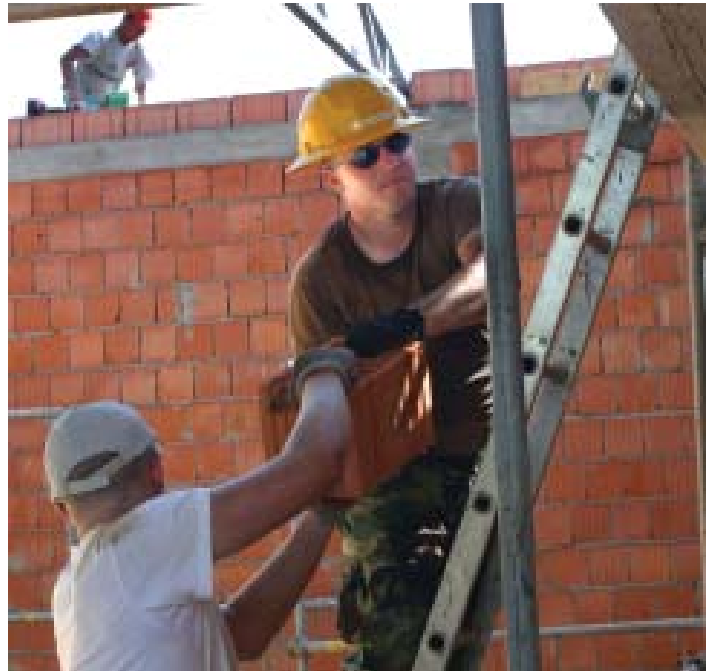
Above: Staff Sgt. Robert Mendez grasps a brick from one of the civilian construction workers at the community center work site while everyone was working to prep the building for the new roof.
